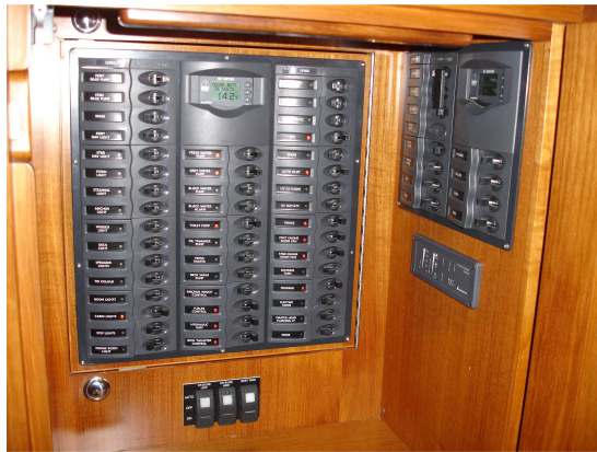
Hidden electrical panel
